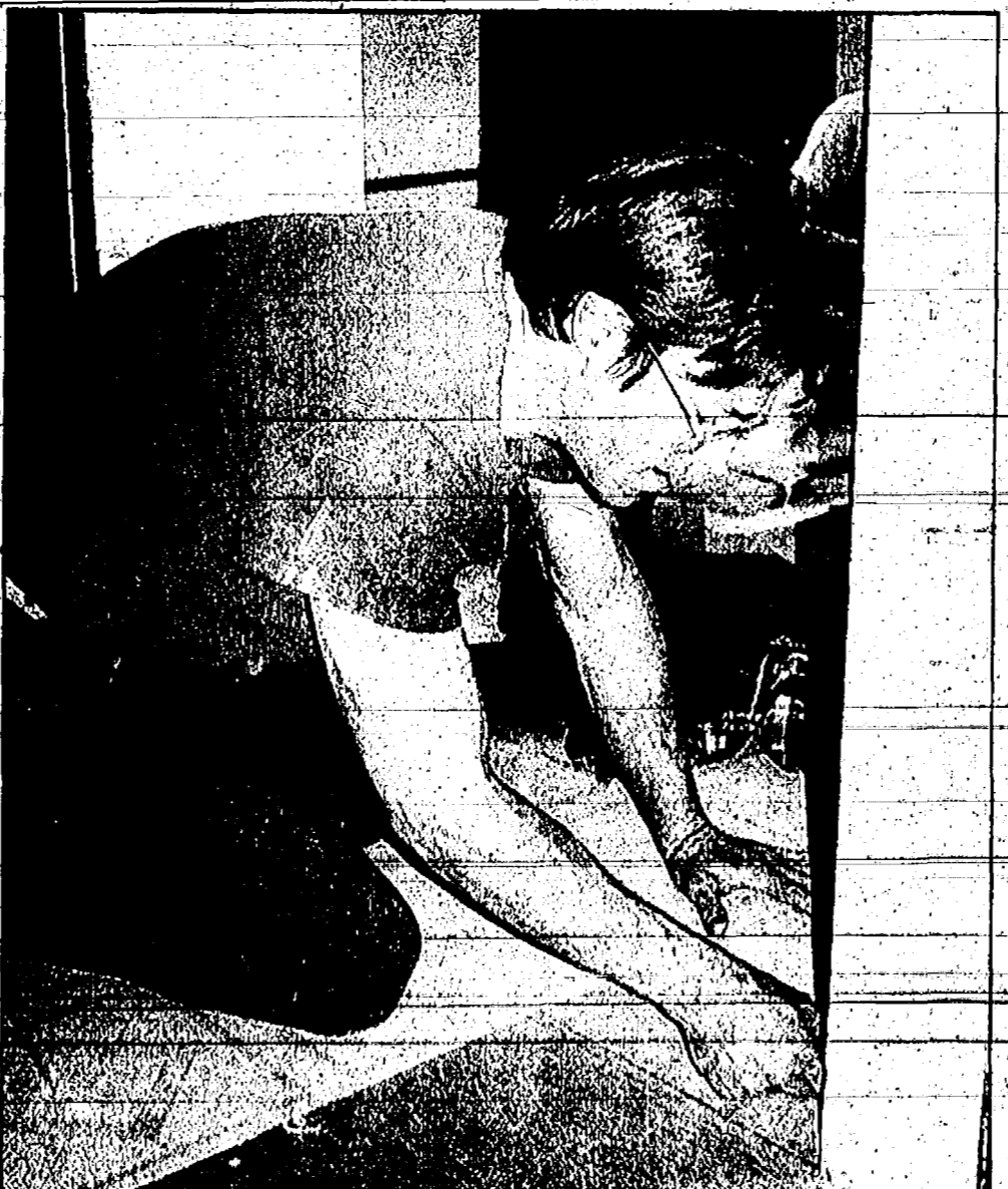
Duane Schroen took a break from making cabinets to rebuild the kitchen floor. He and two other volunteers laid tile on a newly built sub-floor.
